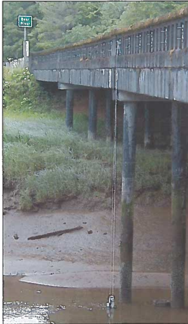
Figure 3-6. Tide gauge deployed at Bear River Bridge
