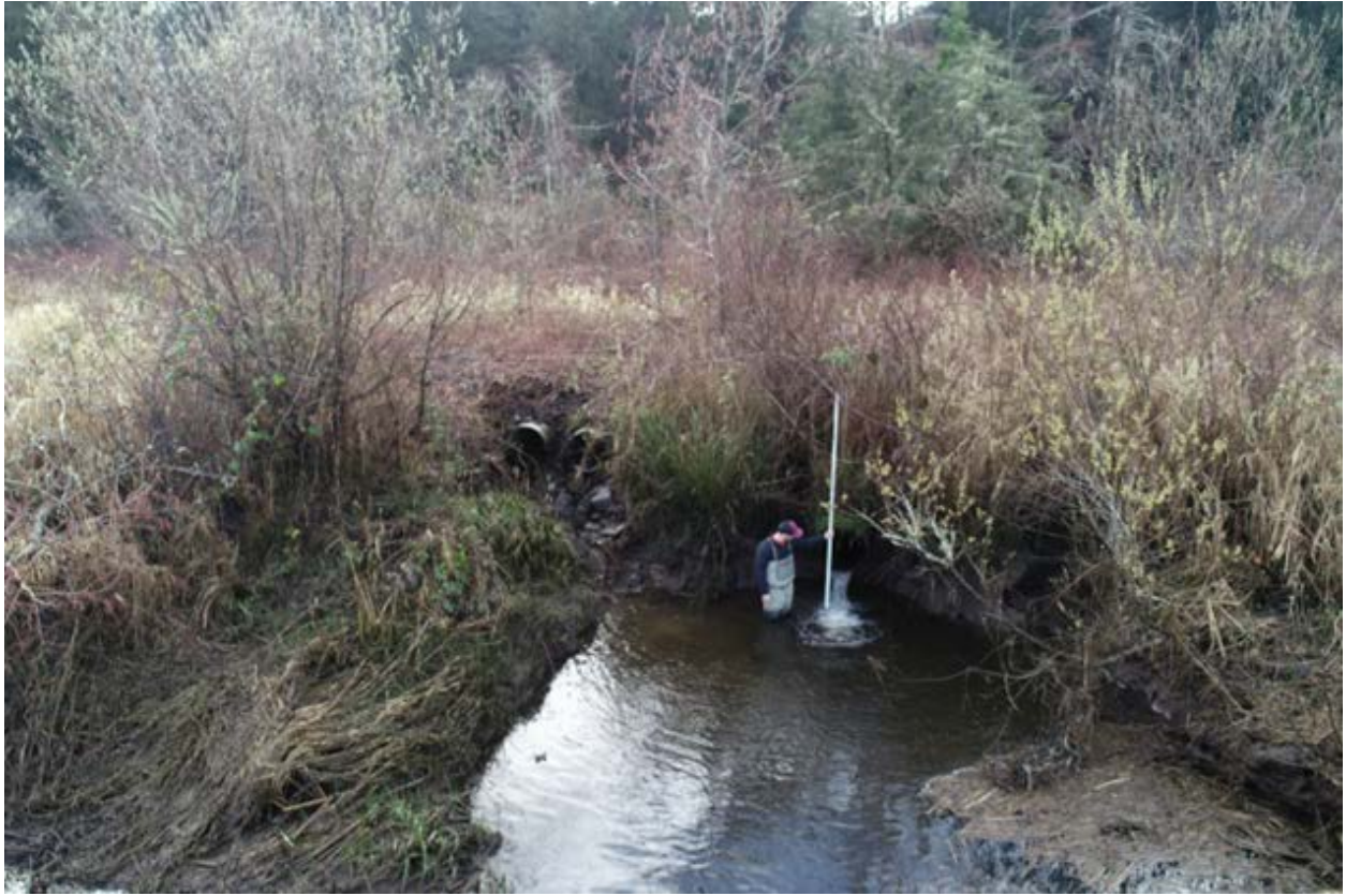
Photo captured from above the existing three small culverts that will be removed and replaced with the single span ~36' bridge.
