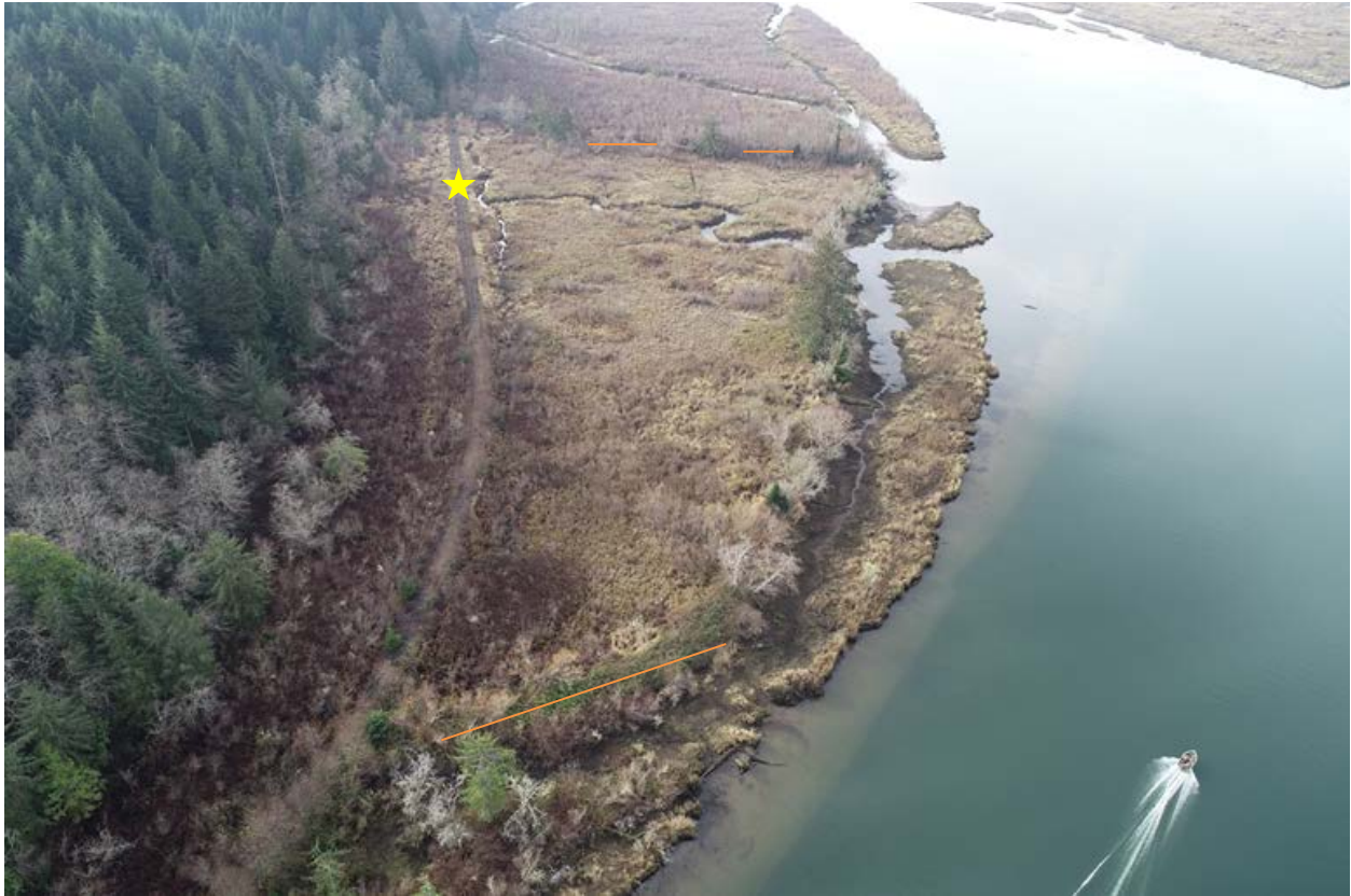
Photo captured from the eastern side of project area, looking to the west. Orange lines indicate the three levee scrapedown areas (Scrapedown A, Scrapedown B, and Scrapedown C). The yellow star indicates the culverts scheduled for removal and the location of the ~36' single span bridge..
